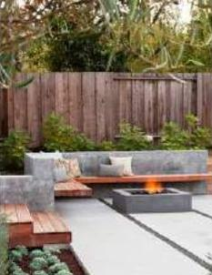
Concrete and timber built-in bench that can act as a retaining wall or garden bed. Timber with a square profile has been used for the seat cantilevered off the concrete.
